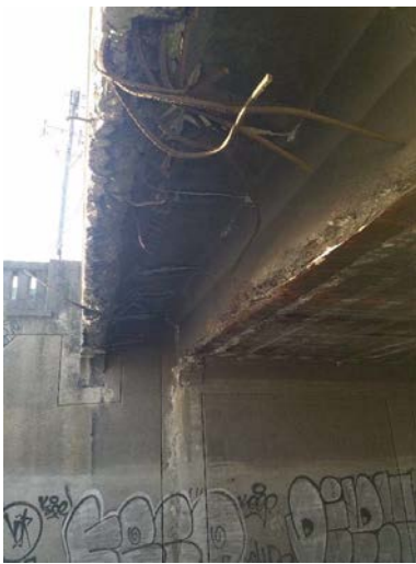
Figure 2: Truck strike damage at bridge
