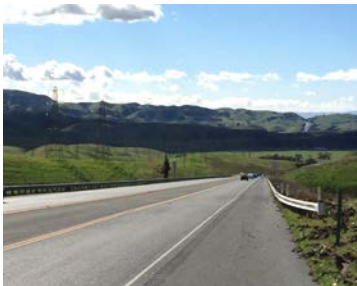
SR-84 looking eastbound near Ruby Hill Road.
