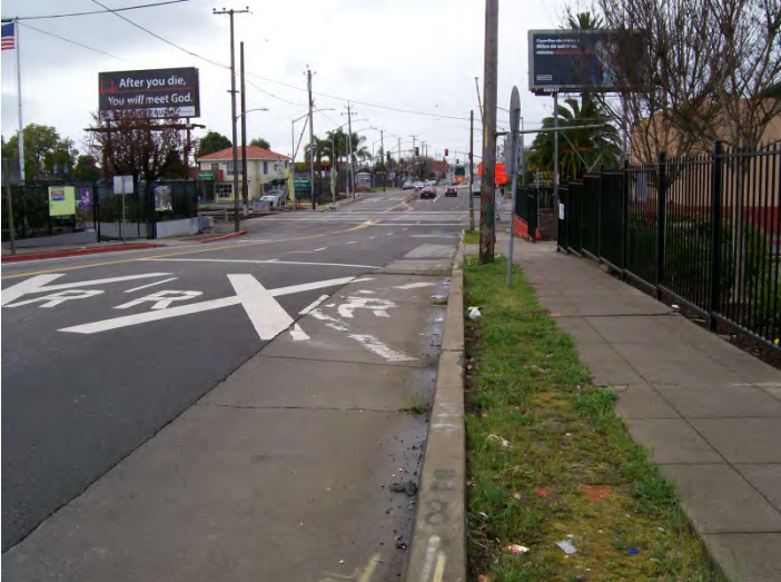
Roadway Looking West
