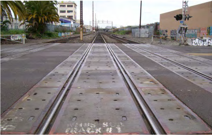
RR Looking North
