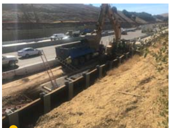
Constructing Drainage System
