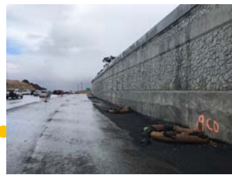
New Pavement in Front of Wall 711
