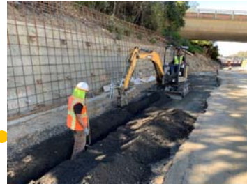
Trenching for installation of conduits and fiber.
