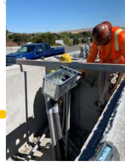
Electrical box installation.
