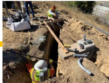
PG&E crew installing meters.
