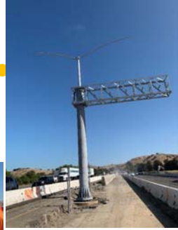
Overhead Sign Structure installation.
