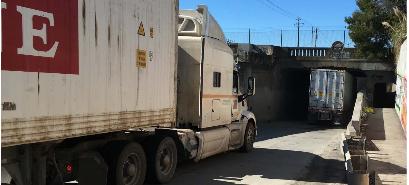
Trucks entering the existing 7th Street underpass to the Port of Oakland.
