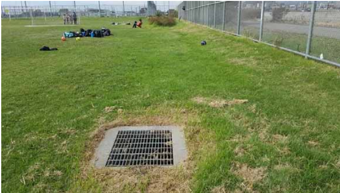
Photo 5. Drainage Grate South of Depression 1, facing north
