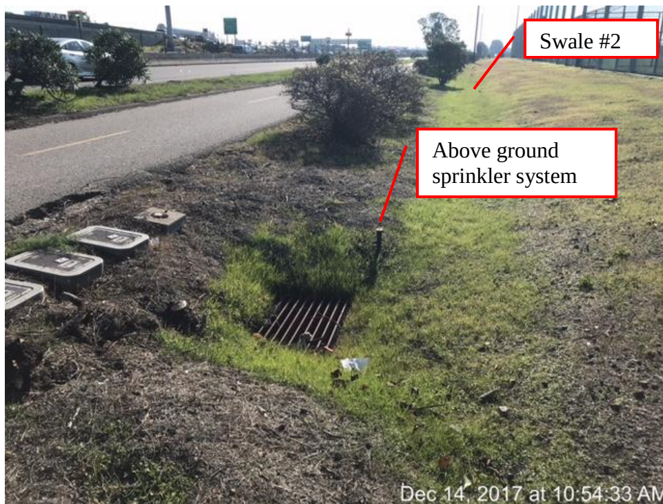
Photo 5. Drainage Inlet along Swale #2, Looking South.
