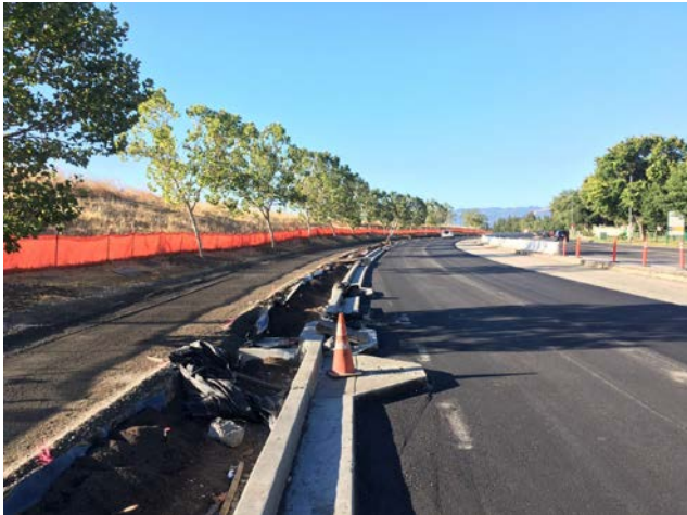
First layer of asphalt paving looking south from Willow Creek.
