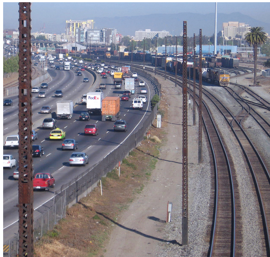
INTERSTATE 880 AND RAIL INFRASTRUCTURE IN ALAMEDA COUNTY
