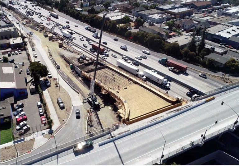
29th Avenue off-ramp under construction, courtesy of Caltrans.
