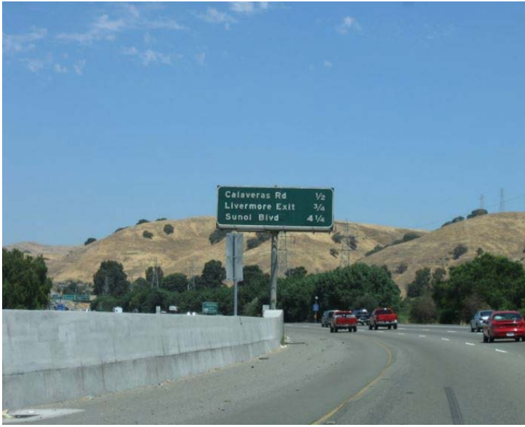
I-680 northbound approaching the Calaveras Road off-ramp.
