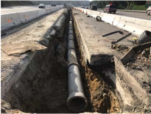
Drainage installation
