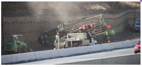
Soil Nail Wall Construction
