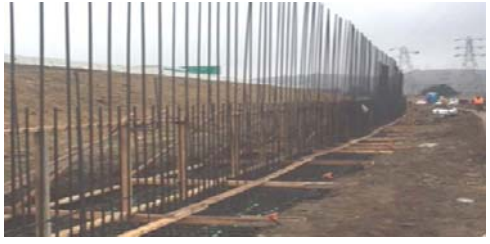
Retaining Wall on Pile Footing
