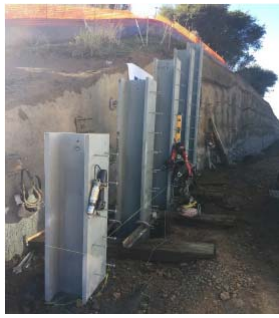
Soldier Pile Wall in progress
