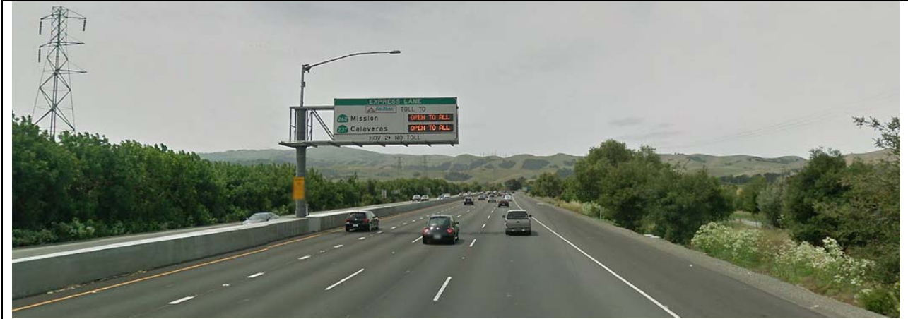
Above: Existing Variable Toll Message Sign (VTMS) on southbound I-680.
