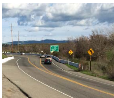
SR-84 Expressway – South Segment.
