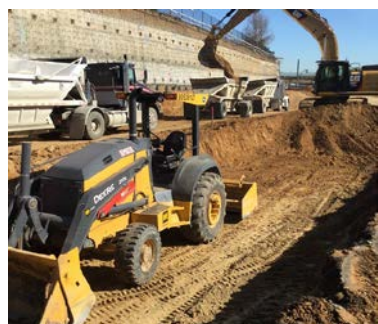
SR-84 Expressway – South Segment.
