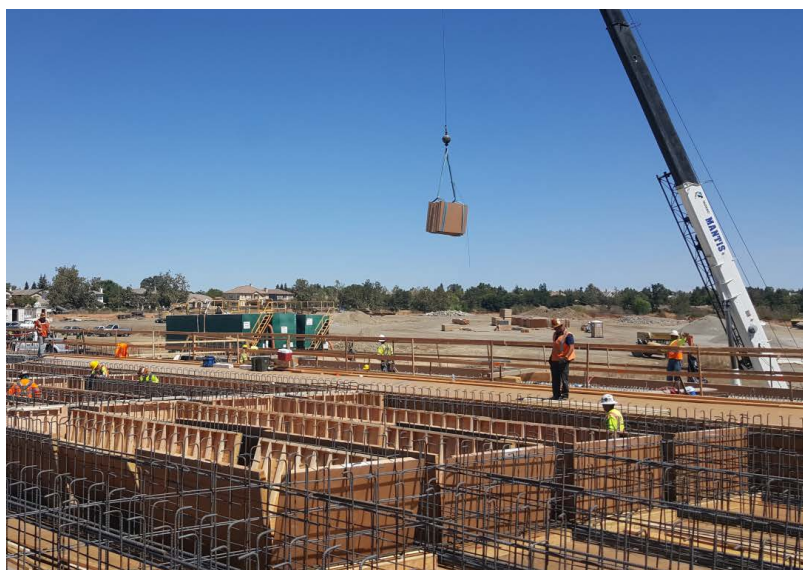
Construction of bridge widening at Arroyo Del Valle.
