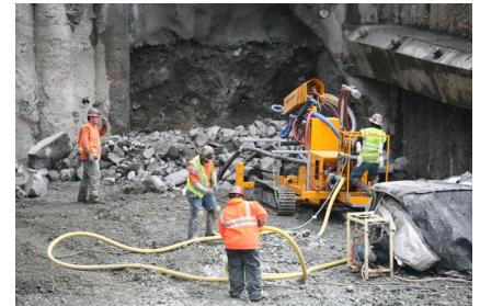
Caldecott Tunnel Fourth Bore Project
