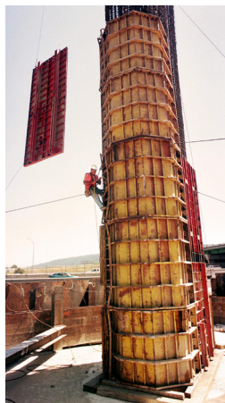
Column Construction on I-580
