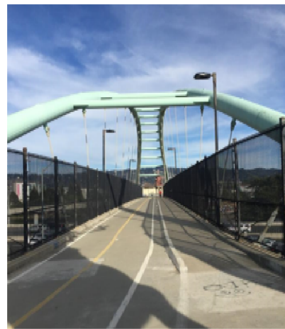
University Avenue bike/pedestrian overcrossing
