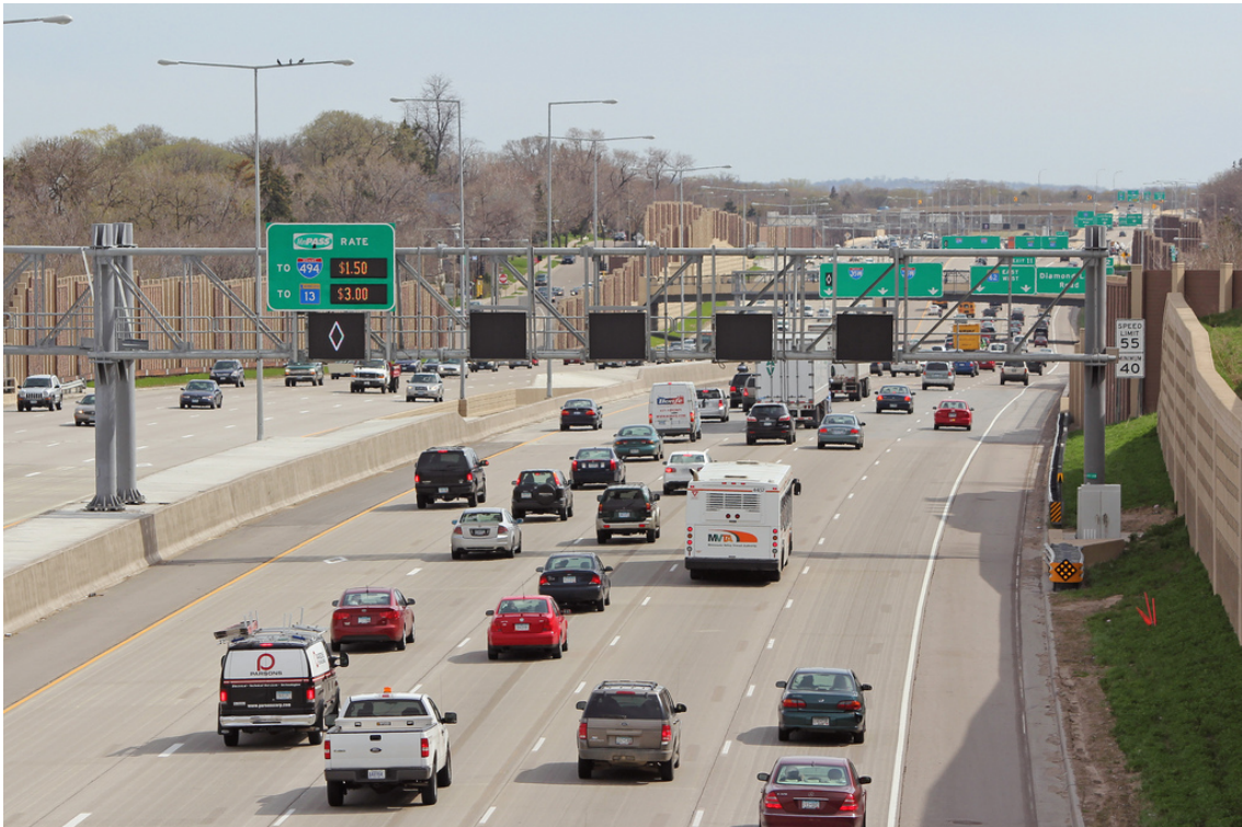
I-35W Express Lane in Minneapolis, Minnesota
