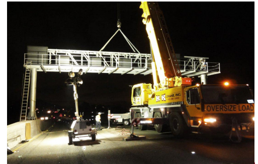
I-80 SMART Corridor Gantry Installation in Berkeley and Emeryville
