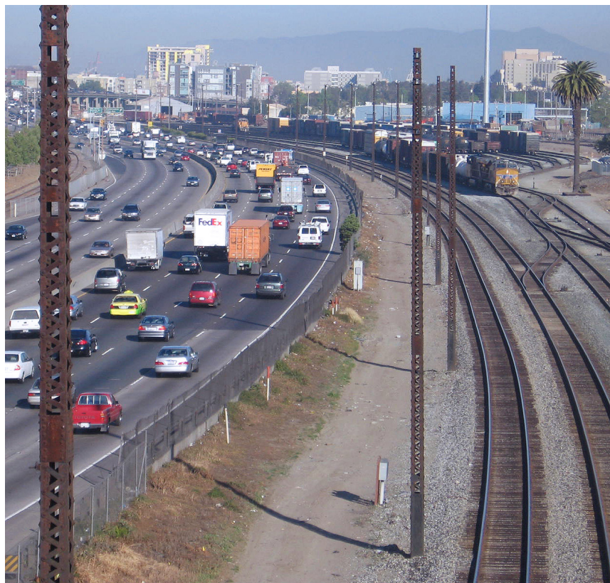
INTERSTATE 880 AND RAIL INFRASTRUCTURE IN ALAMEDA COUNTY
