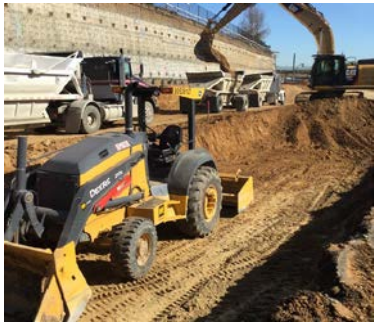
SR-84 Expressway – South Segment.
