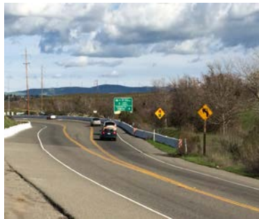
SR-84 Expressway – South Segment.
