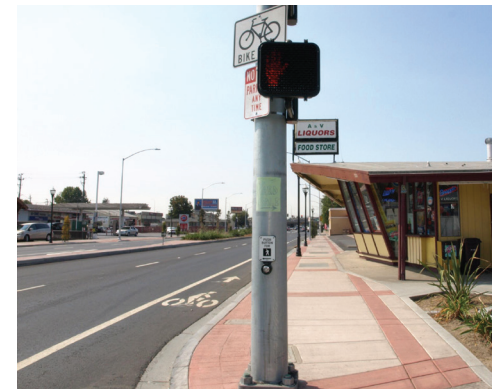
In 2012, Alameda County completed the $32 million Lewelling Boulevard Widening Project, funded by Measure B, which transformed two lanes into a four-lane safe, attractive, less-congested roadway that works for cars, trucks, bicycles and pedestrians.
