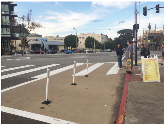
Painted Safety Zone showing parking-prohibited red curb, San Francisco, CA
