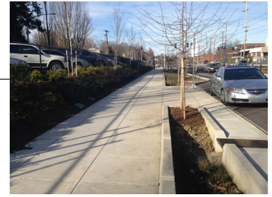
Stormwater planter between sidewalk and street parking
