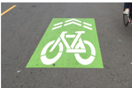
Examples of sharrow markings on the roadway
