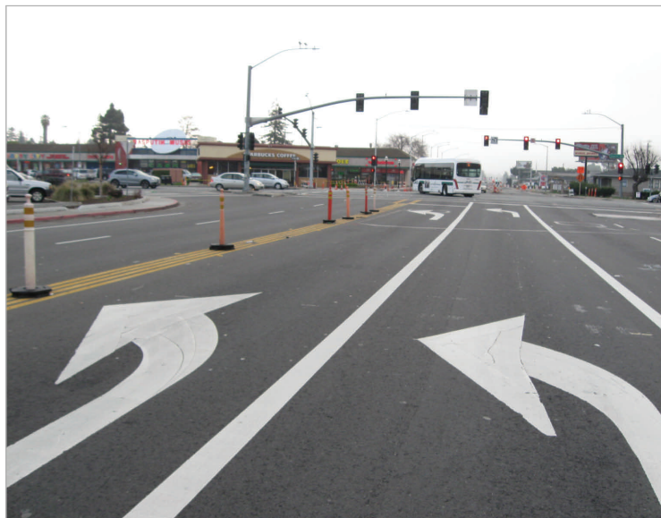
Newly constructed double left hand turn lane on Lewelling Blvd. at the intersection of Lewelling Blvd. and Hesperian Blvd. in San Leandro, CA.
