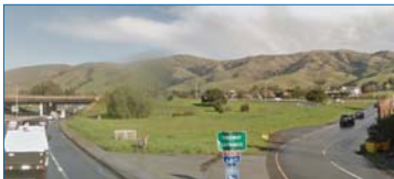
Eastbound SR-262 at the I-680 southbound on-ramp.
