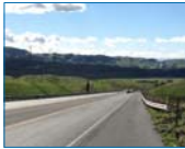
SR-84 looking eastbound near Ruby Hill
