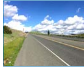
SR-84 looking westbound near Ruby Hill
