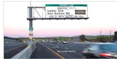
I-580 Express Lanes – Continuous Access
