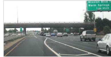
Existing I-680 Express Lanes – Limited Access
