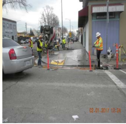
86th St. south-west corner of International Blvd. Curb ramp, sidewalk, gutter, and signal pole foundation construction.
