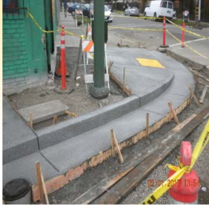
82nd St. south-west corner of International Blvd. Curb ramp, sidewalk, and gutter construction.
