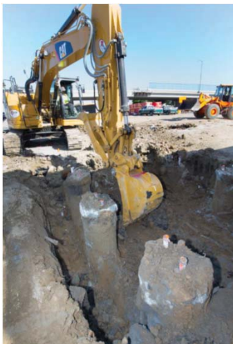
29th Ave. Offramp bridge - Abutment 1 Excavation/completed piles.
