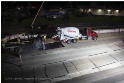
23rd Avenue Overcrossing First stem and soffit pour between Abutment 5 and Bent 3 – June 2018
