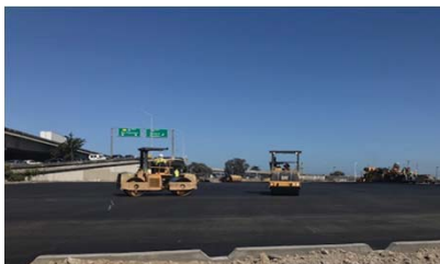
Ancillary Maritime Support Services Truck Parking Area Paving Operation.
