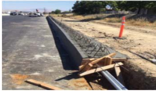
Formed and poured concrete barrier.
