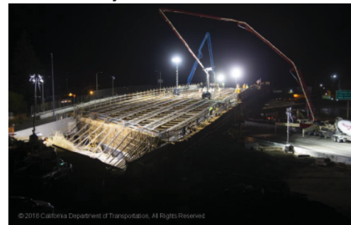
23rd Ave. Overcrossing - 1st Stem and Soffit pour (June 9, 2018).
