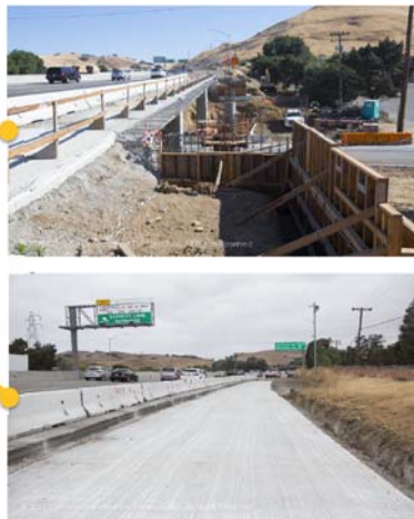
Calaveras Road Bridge Widening
