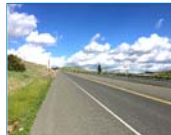
SR-84 looking westbound near Ruby Hill
