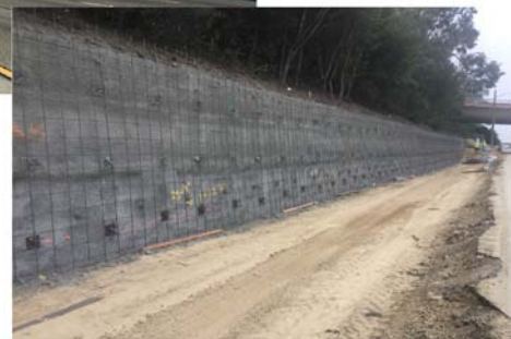
Retaining Wall Construction
