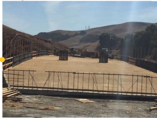
Sheridan Rd Bridge over I-680
