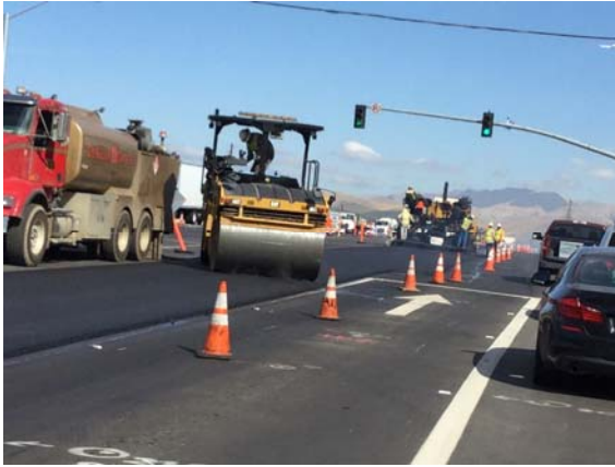
Intersection at Isabel and Concannon: Final lift of rubberized asphalt (October 2018)
