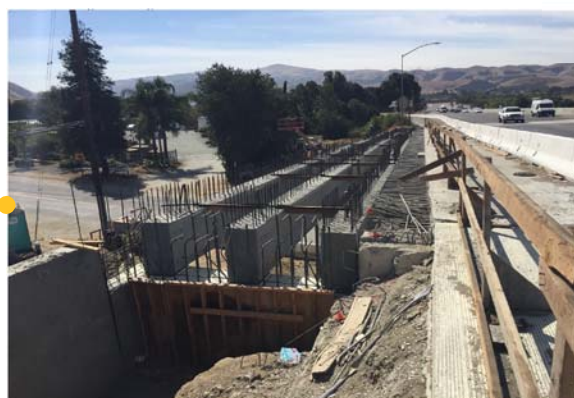
Calaveras Rd Bridge widening
