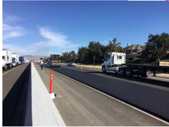
Eastbound Isabel between Vineyard and Concannon: New Rubberized Asphalt (October 2018)
