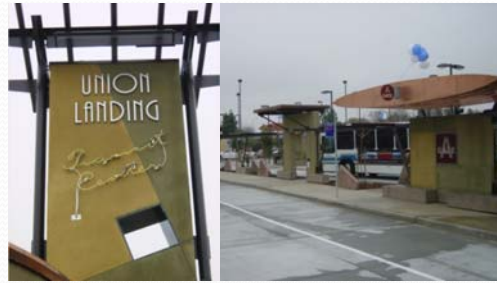
Union Landing Transit Center
