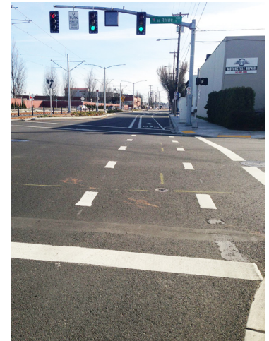
Dotted bike lane marking through street intersection for added bicyclist safety
