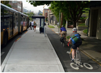
Bus platform with bike lane adjacent to sidewalk Source: NACTO.org
