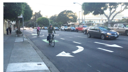
Shared right-turn lane with "sharrow" marking for Class III Bike Routes
