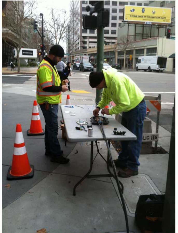
Fiber Optic Splicing - Oakland
