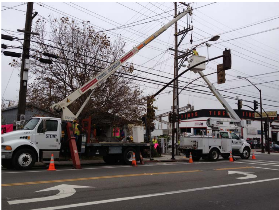
Traffic Signal Modification – 6 th & Gilman
