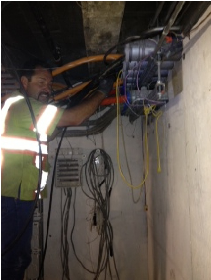
Fiber Installation under Oakland City Hall
