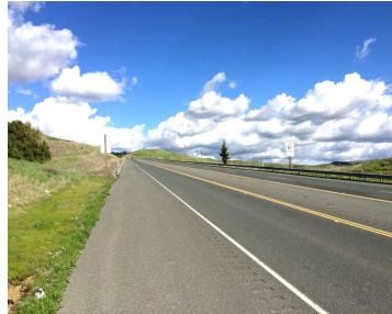
SR-84 looking westbound near Ruby Hill Road.
