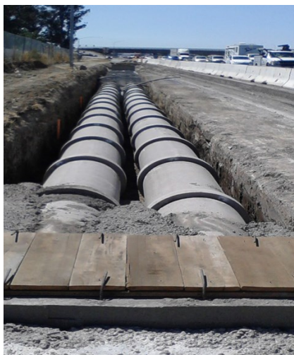
Drainage System #23 (RCP) Installation
