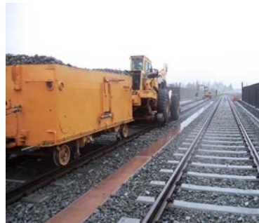
Bay Area BART tracks in construction.
