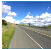
SR-84 looking westbound near Ruby Hill
