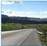
SR-84 looking eastbound near Ruby Hill
