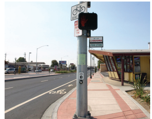
In 2012, Alameda County completed the $32 million Lewelling Boulevard Widening Project, funded by Measure B, which transformed two lanes into a four-lane safe, attractive, less-congested roadway that works for cars, trucks, bicycles and pedestrians.
