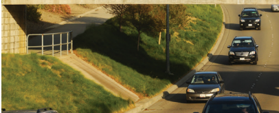
Measure B funds operations and Alameda County's share of station improvements for the Altamont Commuter Express Rail. Signal system upgrades, a new maintenance facility, purchase of additional rolling stock and other improvements are funded by Measure B sales tax dollars.
