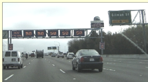
(left) I-80 ICM project corridor; Aerial of I-80 looking South. (top middle) Mainline I-80 and (top right) San Pablo Arterial. (bottom right) Example of overhead lane use signs and variable advisory speed signs on WB I-80 from Cutting St. to Powell St.
