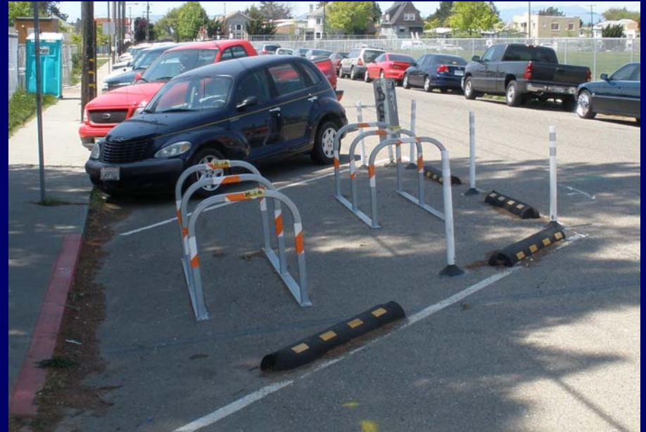
Diagonal Parking: In-street bike parking delineated by pavement markings or rubber curbing on asphalt
