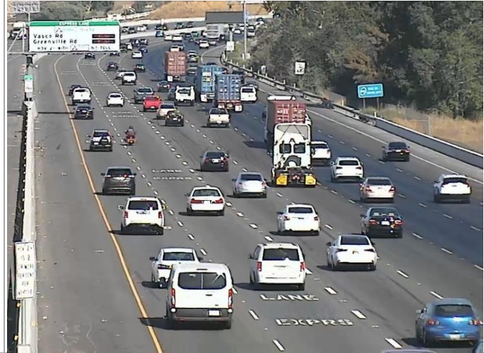
Two-Lane Continuous Access
