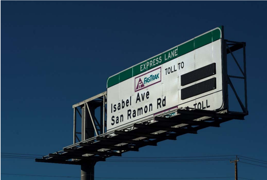
Figure 3: I-580 Westbound Express Lanes Toll Gantry Sign
