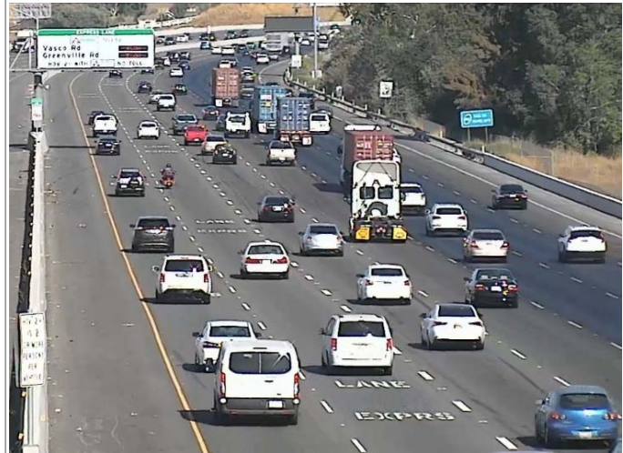
Two-Lane Continuous Access
