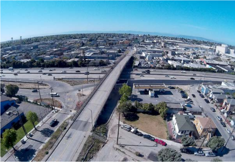
Pre-demolition of the 29th Avenue overcrossing, courtesy of Caltrans.
