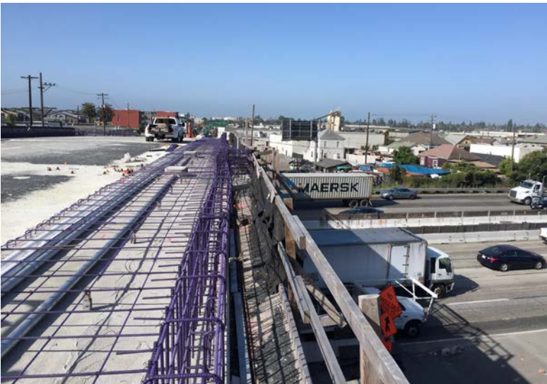
Nearly completed 29th Avenue overcrossing, courtesy of Caltrans.
