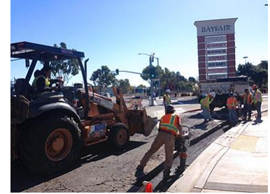
Accessible Pedestrian Signal Upgrade
