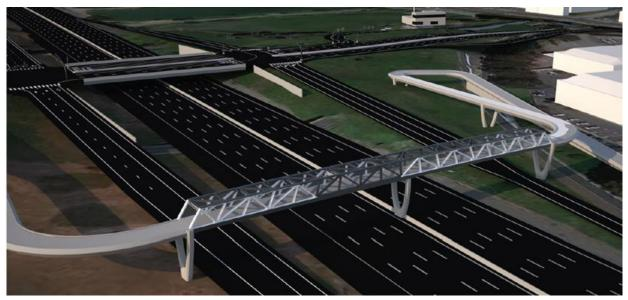
Figure 1.5-25 Truss Design Option
