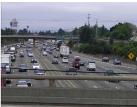
View of I-880 at Marina Blvd. overcrossing looking north.
