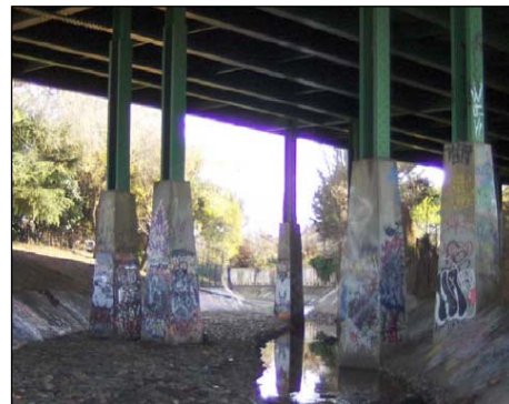
I-880 Bridge footings at San Leandro Creek.
