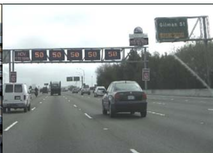
Left: I-80 mainline in Berkeley, CA.
