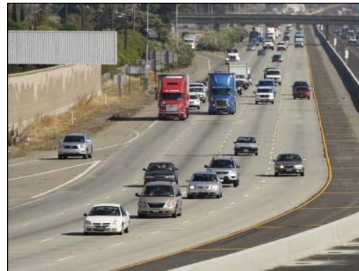
Westbound I-580 Corridor (looking east); the HOT lane Environmental Phase began August 2011.
