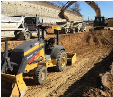
SR-84 Expressway – South Segment.
