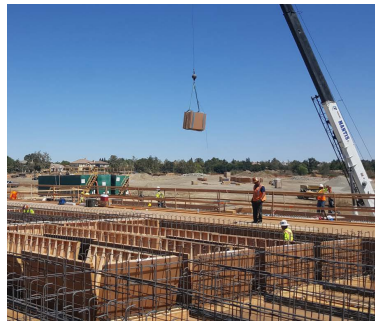
Construction of bridge widening at Arroyo Del Valle.
